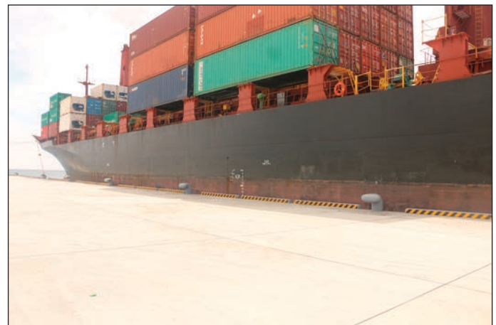
SIPA's new $190 million wharf was officially opened on 10th October, 2016. This Japan funded project will boost Solomon Islands international trade in goods. [Photo supplied by Solomon Star]
